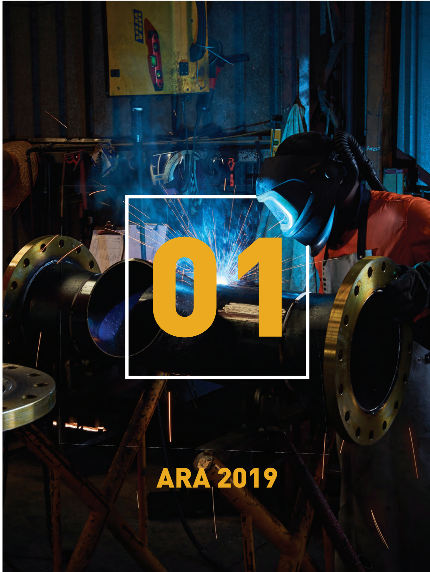
Photograph Pipe Fabrication, ARA Fire.
