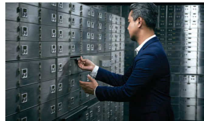
Photographs Top left: NEDA facility services team. Top right: GME manufacturing facility - Victoria. Bottom right: GME manufactured Cryoquip container. Bottom left: ARA Vaults safety deposit boxes - Bella Vista.
