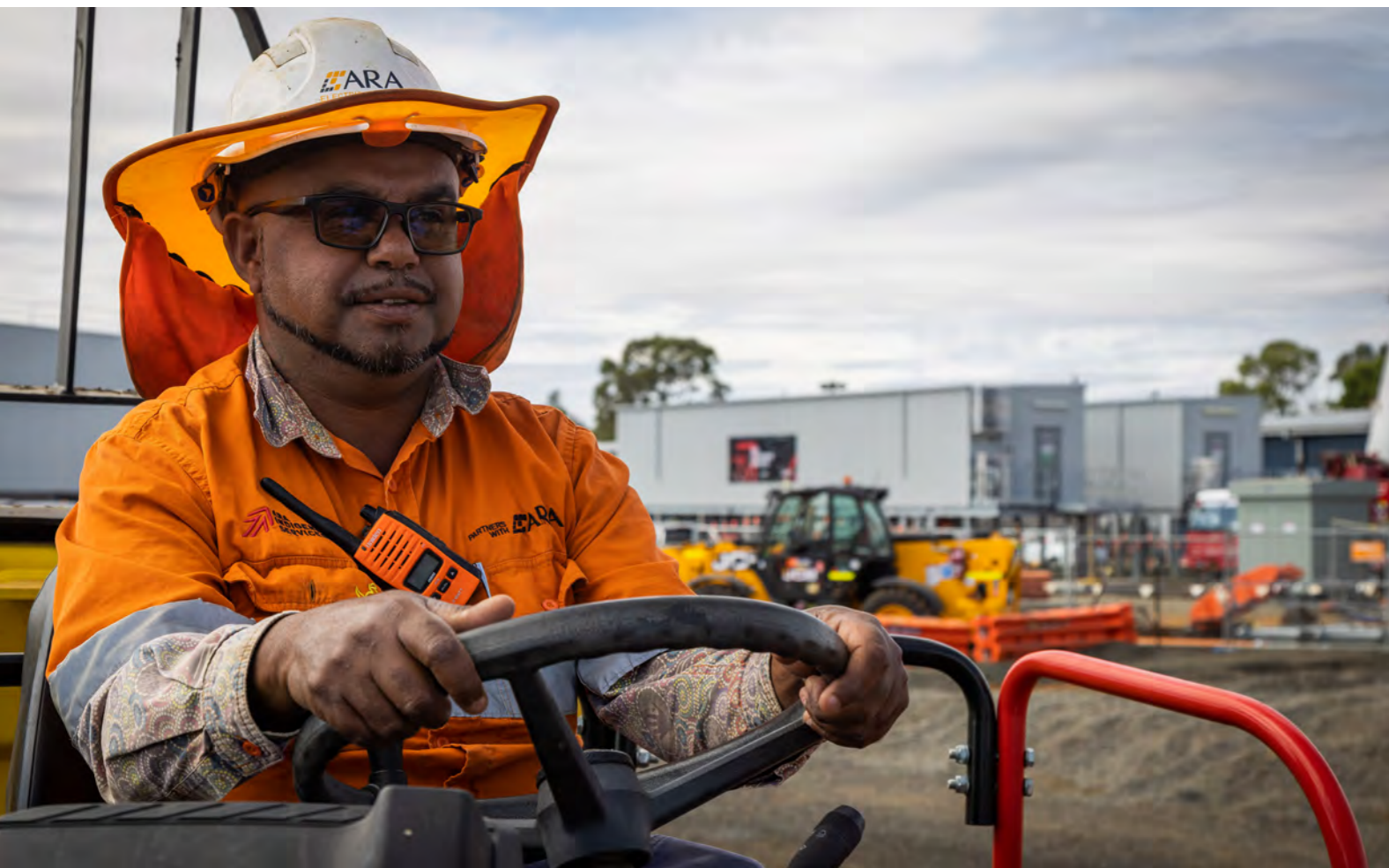
Photograph ARA Indigenous Services switchroom installation, Dubbo NSW
